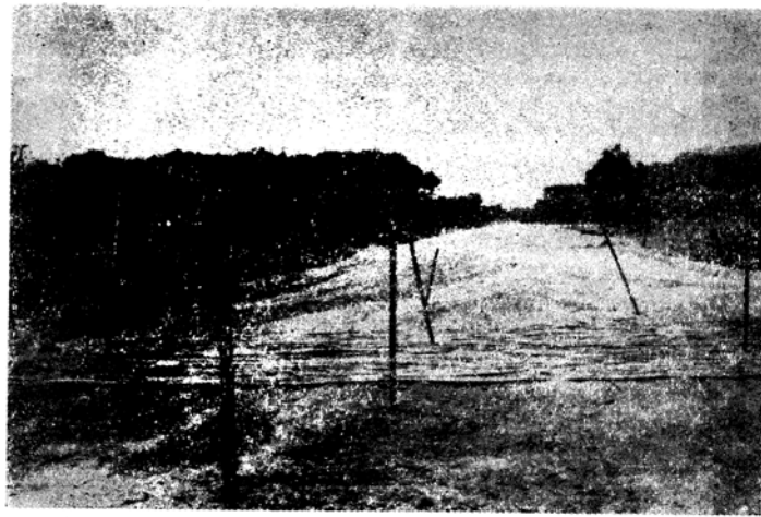
Fig. 7 Second Layer Fascines
